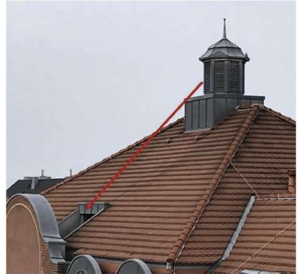
Figure 4. Exhaust air opening in the tower at the highest point of the roof building of the nursing home as well as the location of the supply air opening (red arrow).
