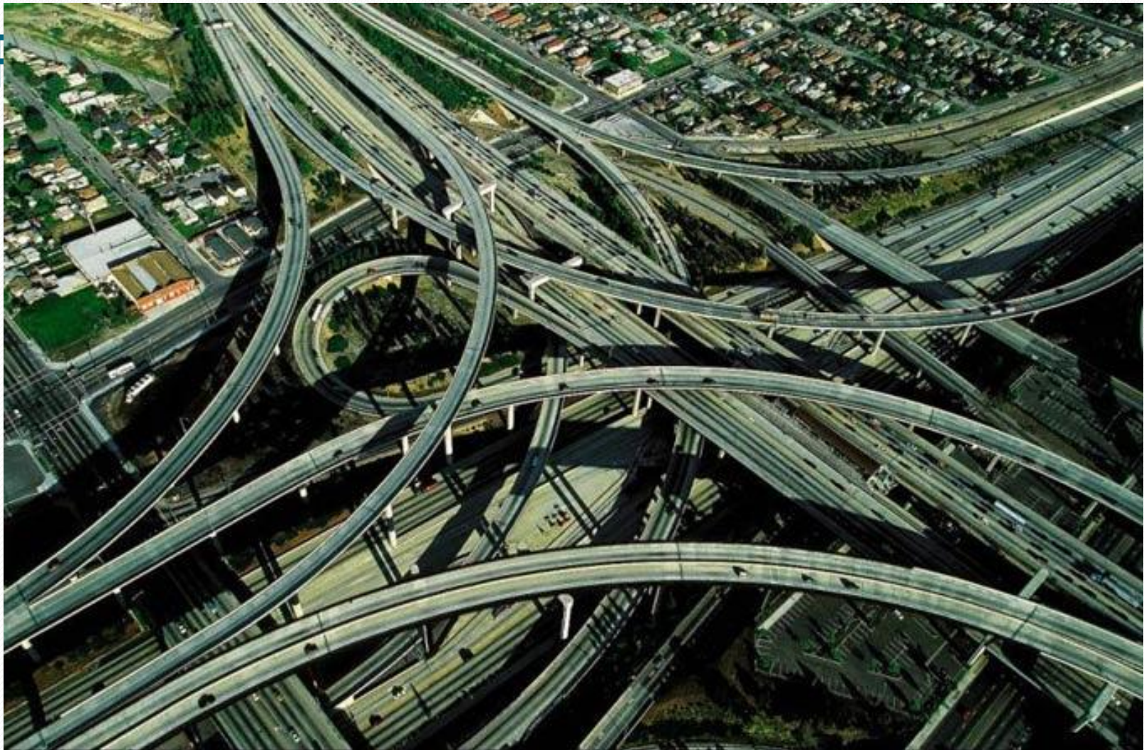
INTERCHANGE BETWEEN THE 5 AND 110 FREEWAYS, Los Angeles, United States (N 34°02' - W 118°16') http://www.gannarthusbertrand.org
