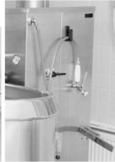
Fig. 3. (a) Hydrotherapy Tub and hand held shower. (b) Close-up of the hand held shower.
